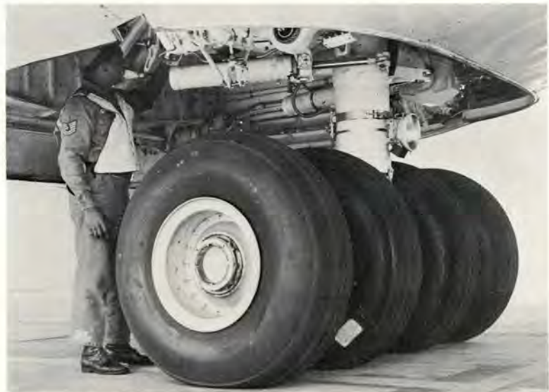
Quick Service Maintenance NCO installs nose gear pin.
